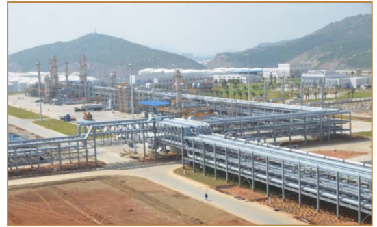
Onshore gas terminal
