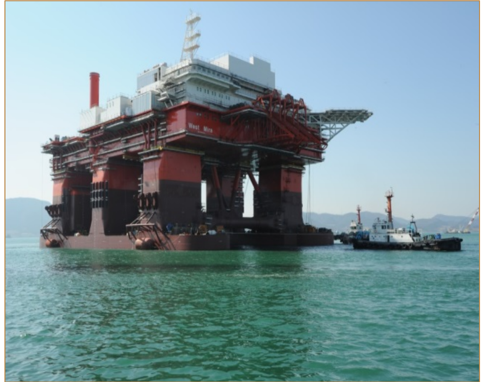
West Mira under construction
