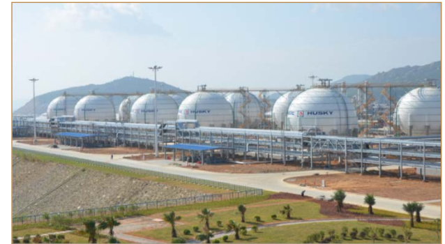
Onshore gas terminal
