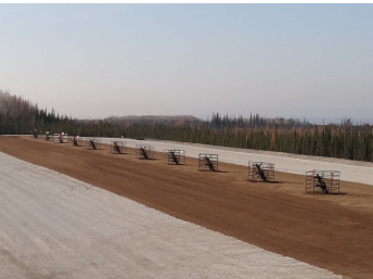
Completed Pad G
