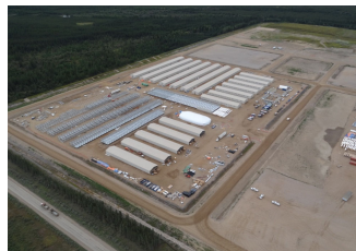
Camp construction underway
